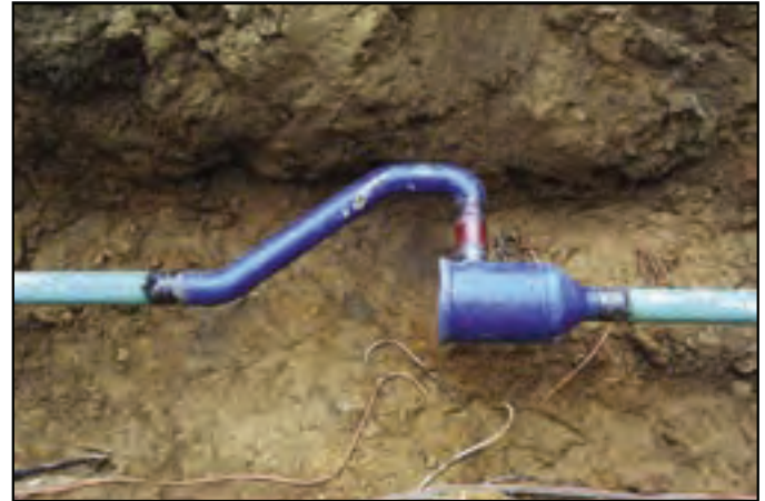
Appalachian Basin VortexFlow™ SX Gathering Line Installation with Spool
