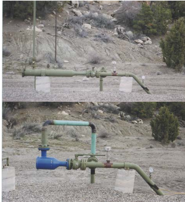
4 Inch Line Pig Launcher Replacement
